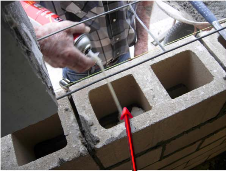
fill wall with foam to insulate
