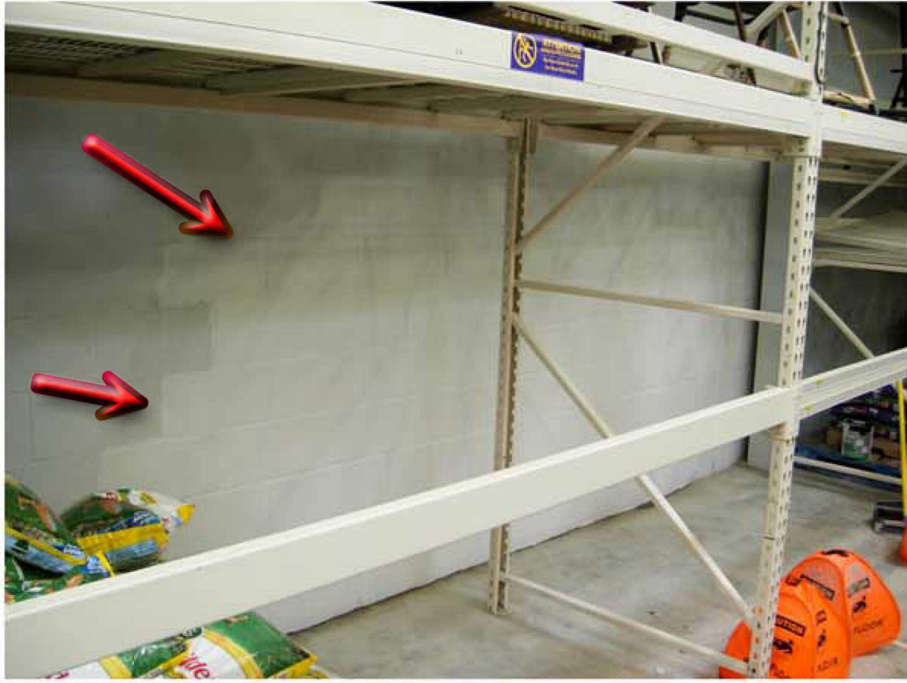
Wall repair done
